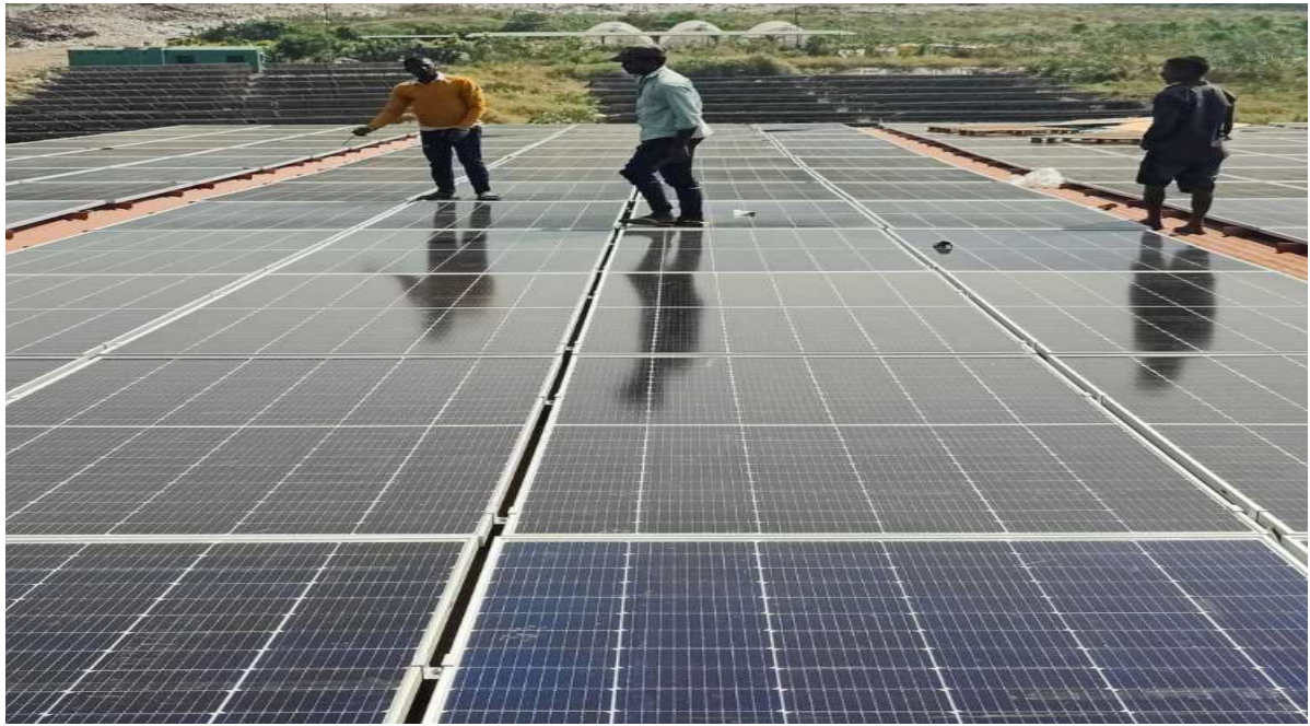
Pic. 3: Installation of 1504 KW Solar Power System on Compost Depo for Satara municipal council
