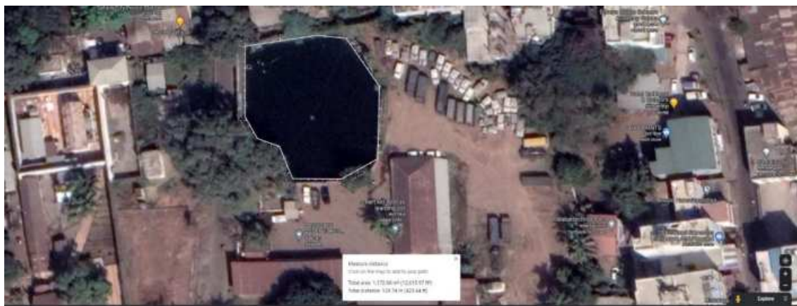
Pic. 18: MT Tank
