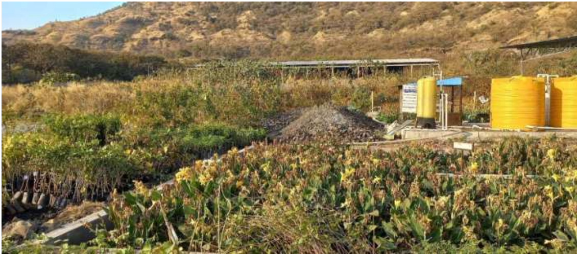
Pic. 6: Biomining at Soangaon waste management depot
