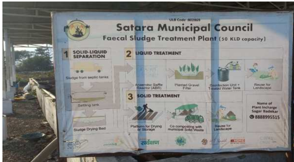
Pic. 1: Sludge treatment plant at Saogaon
